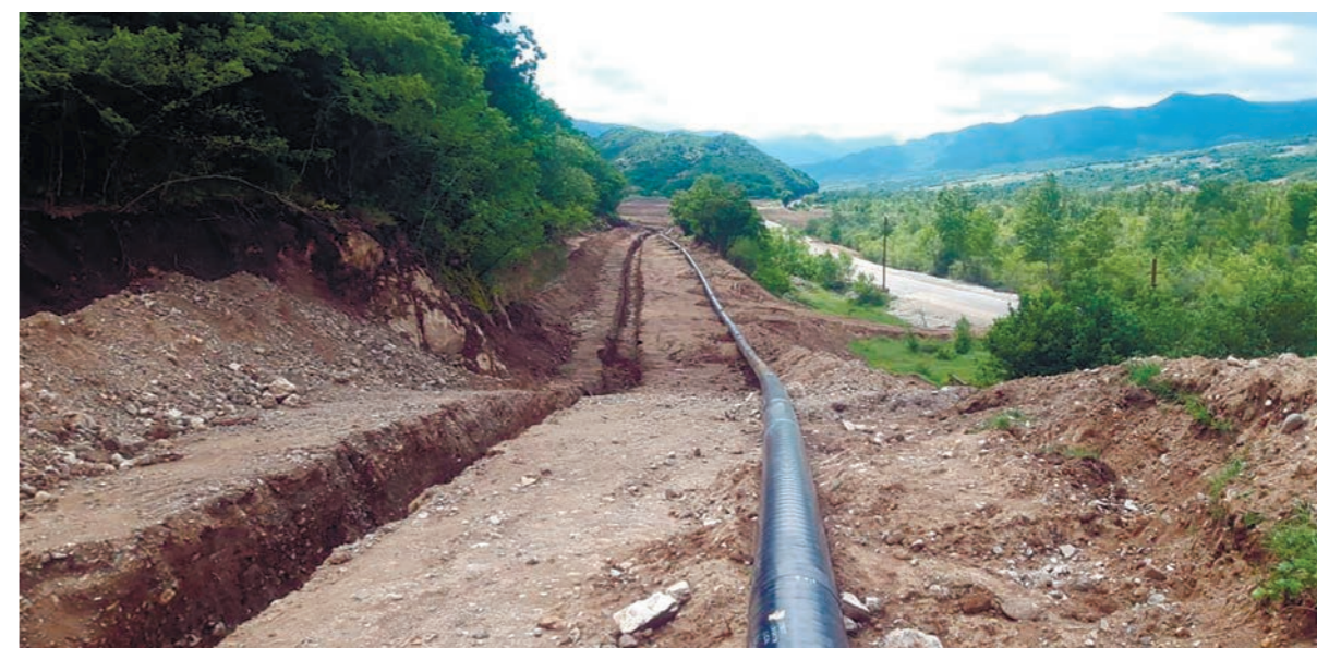
Figure VI.1. Laying of Agdam-Kalbajar gas pipeline
