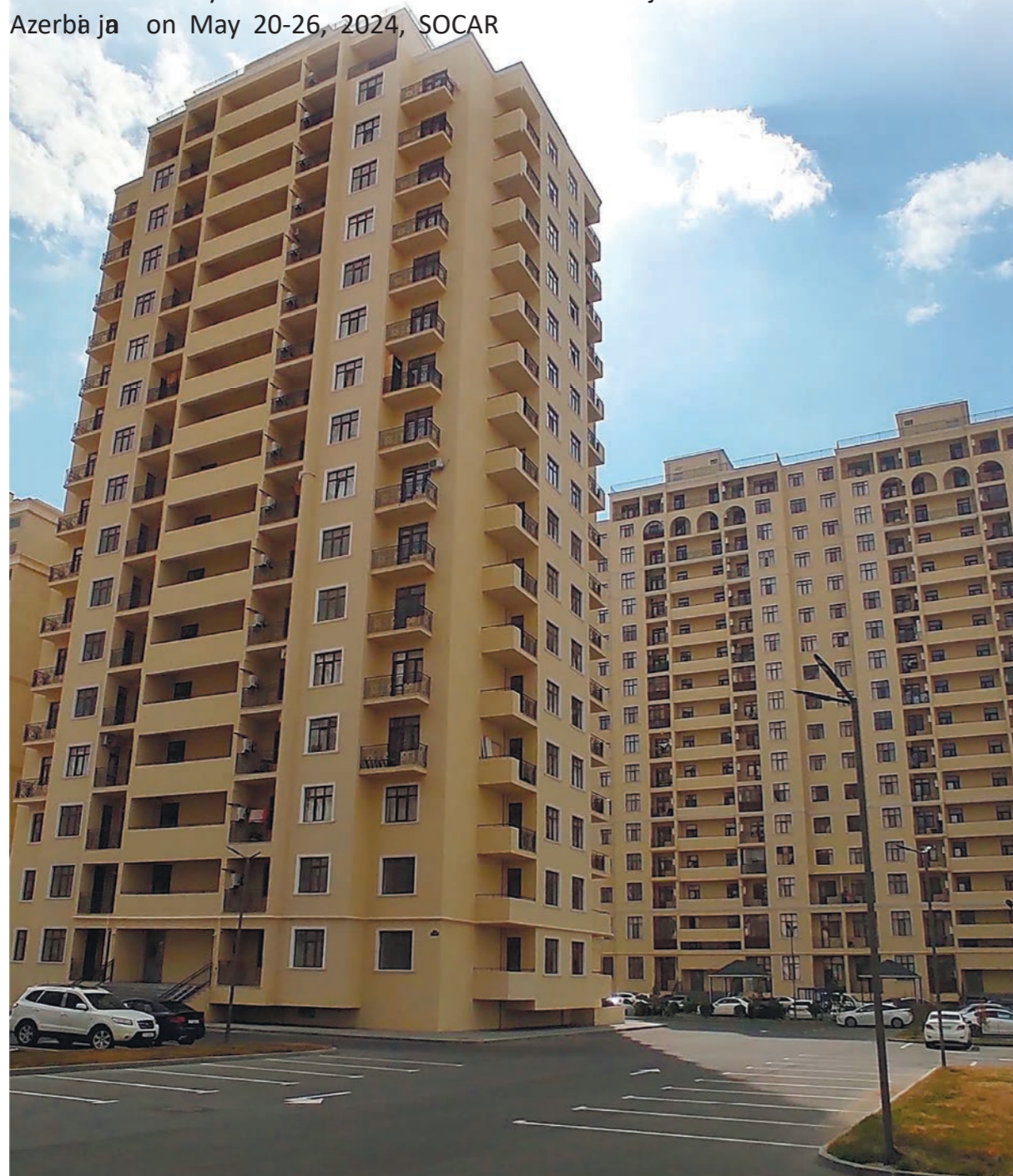
Figure XVIII.1. New residential complex constructed for oil engineers
