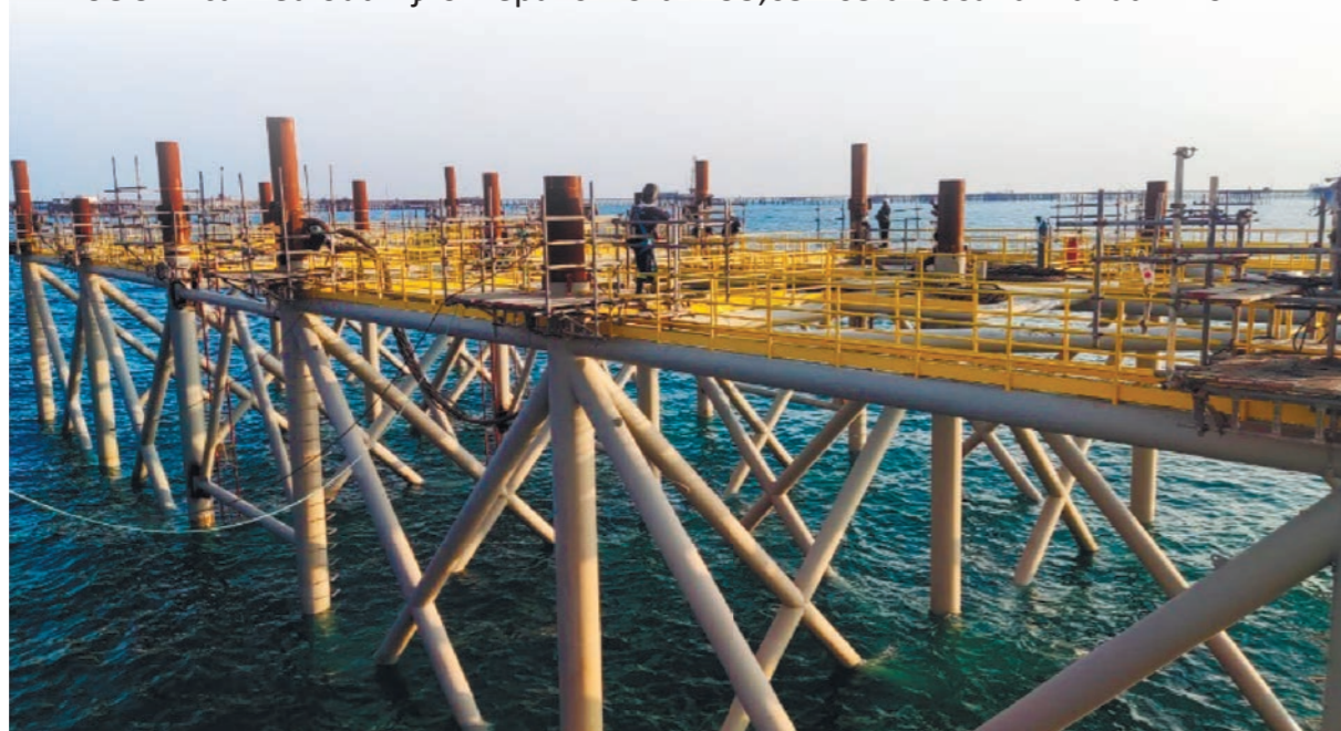
Figure X.1. Construction of jacket 2345 in "Neft Dashlary"
